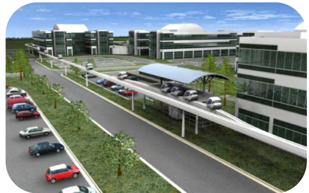
Figure 11. Typical elevated station
