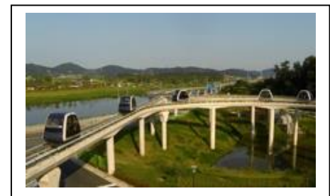
Figure 27 - Pre-cast concrete to withstand earthquakes and severe weather, and secured over marshland; hence, structure is larger than normal.
