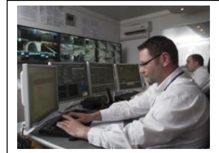
Figure 17 - Heathrow Control Room.
