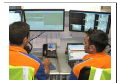
Figure 24 - Masdar Control Room.
