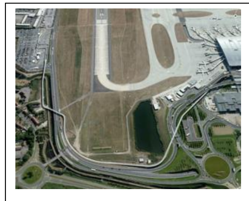
Figure 13 –Aerial view of the Heathrow track from the parking lots on the left to Terminal 5 on the right.
