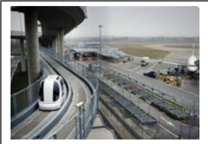
Figure 14 - Vehicle running under Access Road.
