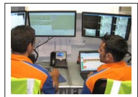
Figure B-12: Masdar Control Room.
