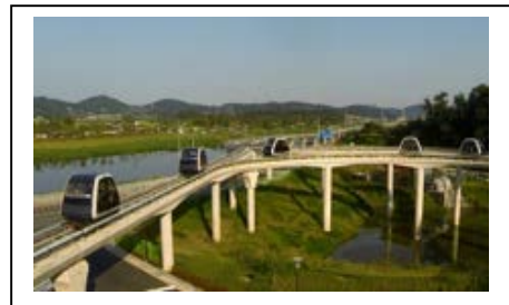
Figure B-15: Pre-cast concrete to withstand earthquakes and severe weather, and secured over marshland; hence, structure is larger than normal.
